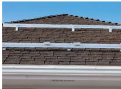
SolarEZ rails minimize roof penetrations.
